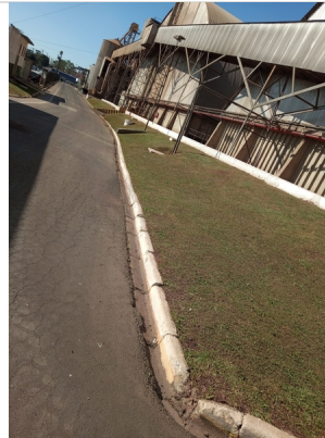
Silo 1 e 2 ok
